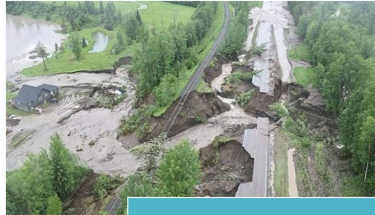
Rail and Highway Access
