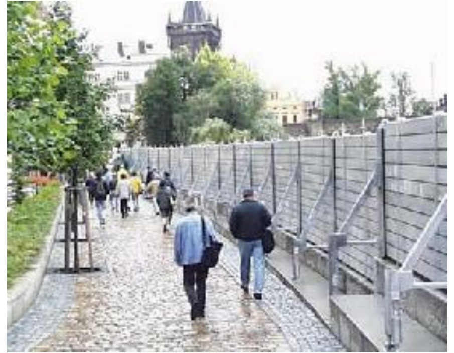
Temporary Flood Wall
