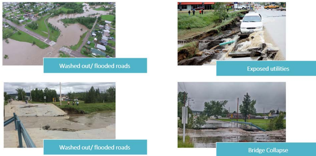
Figure 11: Examples of direct flood impacts in Dawson Creek
