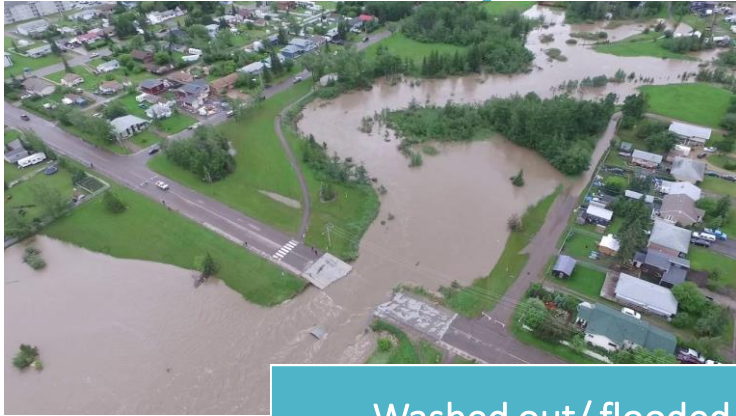
Washed out/ flooded roads
