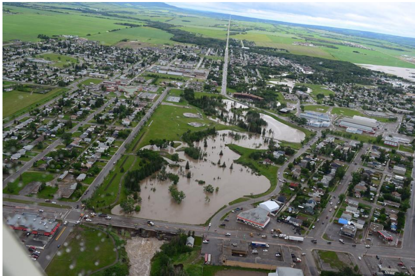
Figure 6: Photo of Flooded Dawson Creek in June 2016
