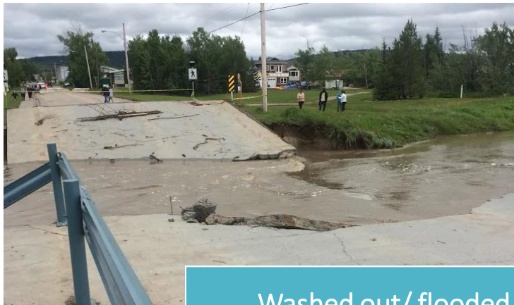
Washed out/ flooded roads
