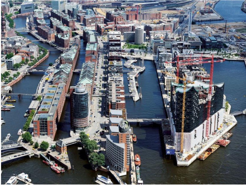
Raising Critical Infrastructure
