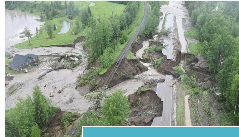
Rail and Highway Access
