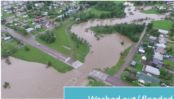
Washed out/ flooded roads
