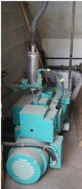
Figure 12: Standby Generator
