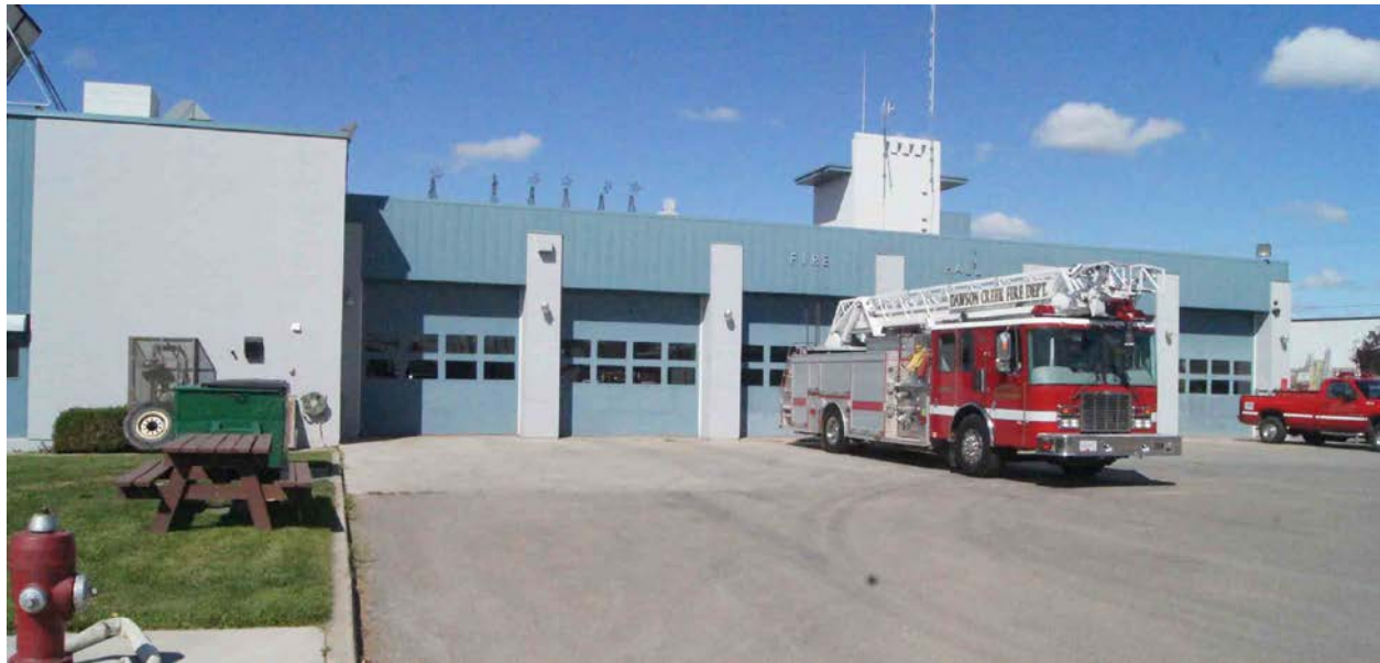
Figure 19: Dawson Creek Fire Hall
