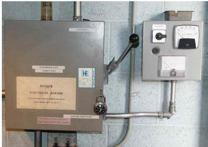
Figure 13: Transfer Switch
