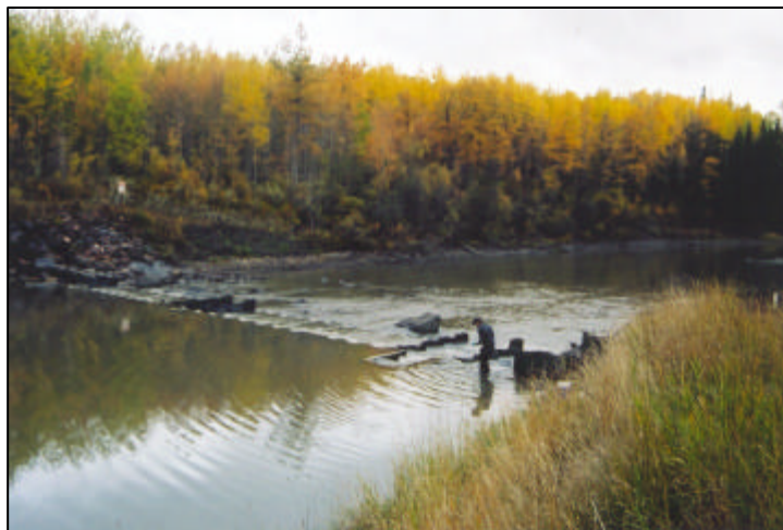
Plate 2. Cross-stream weir located immediately downstream of the Arras pump house. The weir raises water levels to ensure that there is sufficient water to support domestic users (October, 2002).
