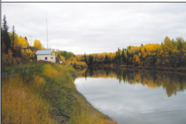
Plate 1. An upstream view of the Kiskatinaw River (from the cross-channel weir) and the Dawson Creek pump house.
